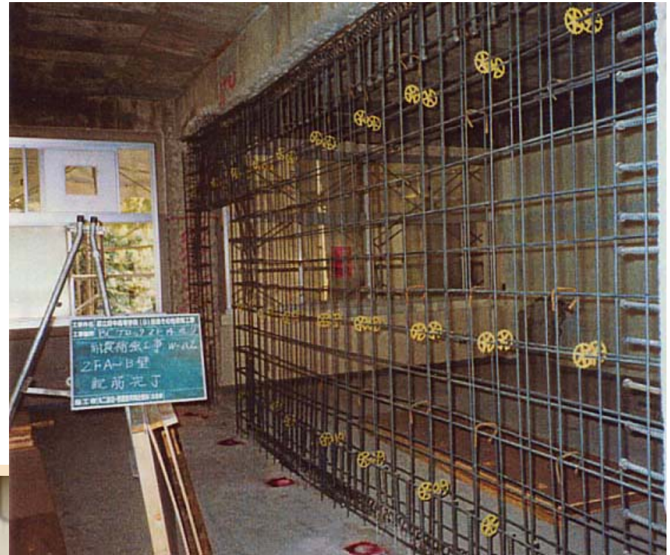
Extension of Infill RC Wall
