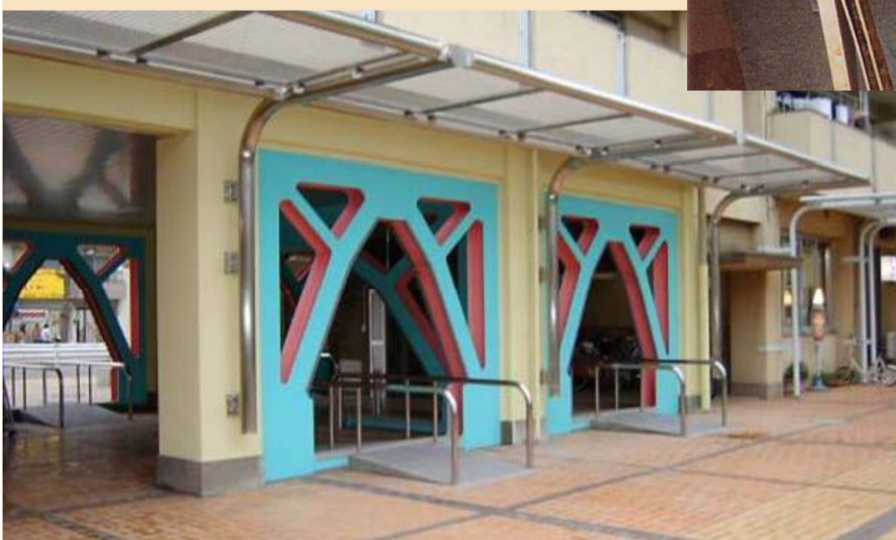
Extension of Infill Steel Brace
