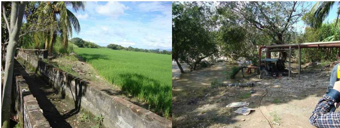
Fig. 8.3.2-3 Channels and Water Pumps for Irrigation in Irrigation Areas Upstream Neiva
