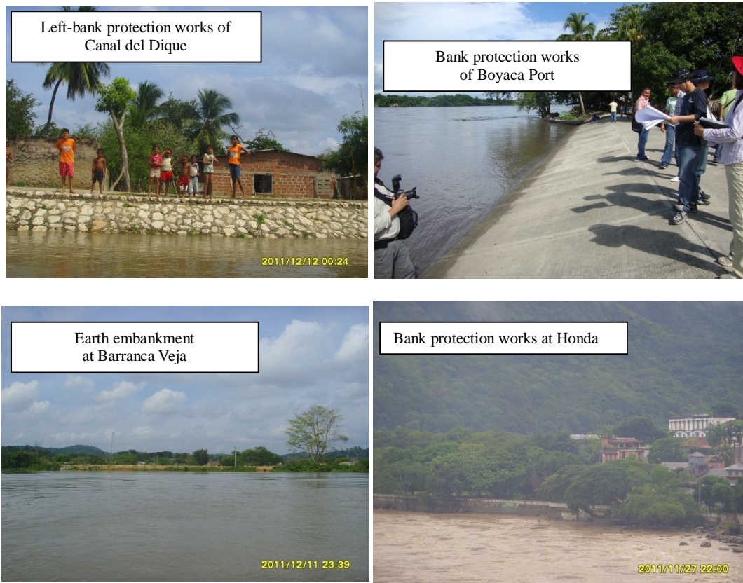
Fig. 7.3.2-1 Photos of Typical Bank Protection Works Scattered along River Bank
