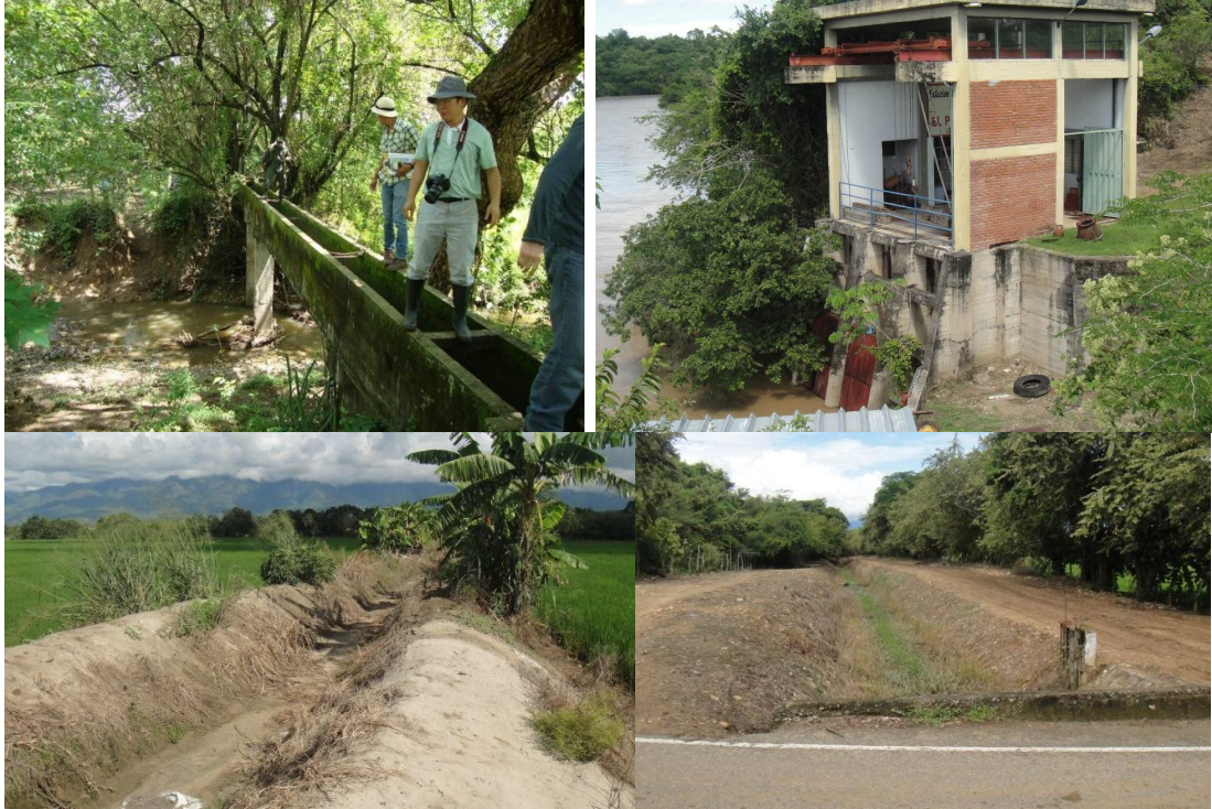
Fig. 8.3.2-4 Aqueduct, Irrigation Pump Station, Channel and other Irrigation Facilities of Irrigation Areas near Villavieja
