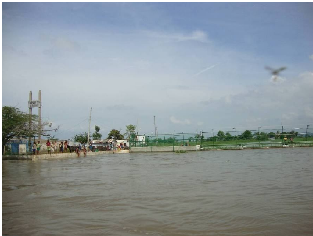
Fig. 8.3.2-5 One of the Gates of Guajaro Irrigation Reservoir at Entrance of Dique Canal
